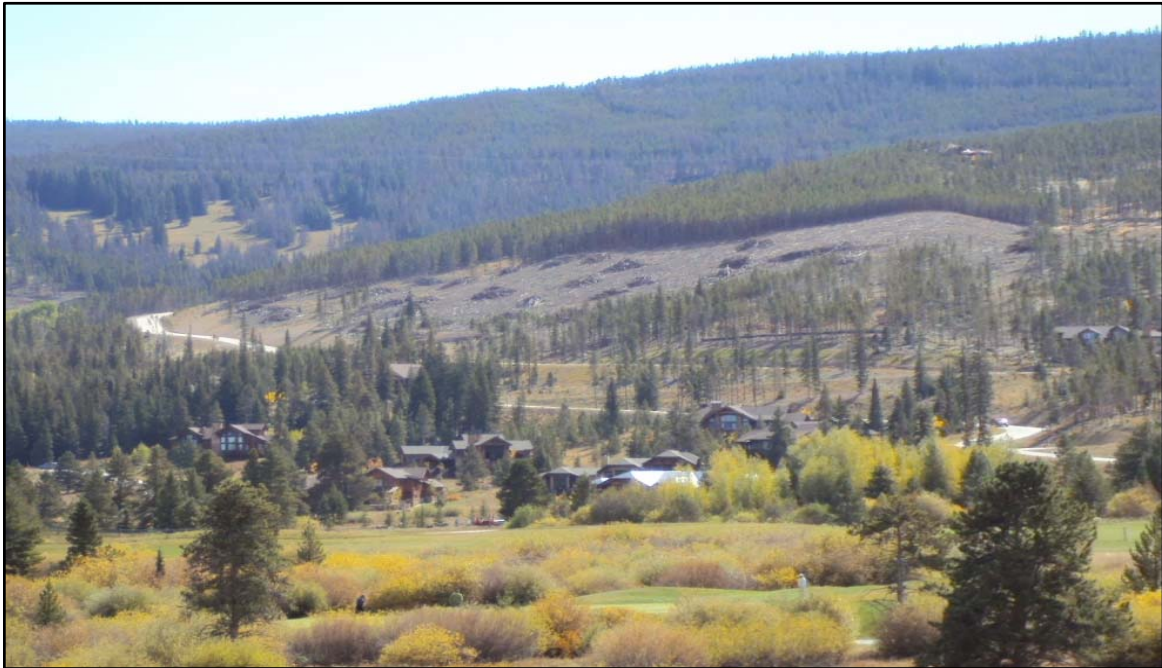
Fuel breaks have been created throughout many areas in Summit County to push the forest back from homes. Beetlekill trees were removed.
