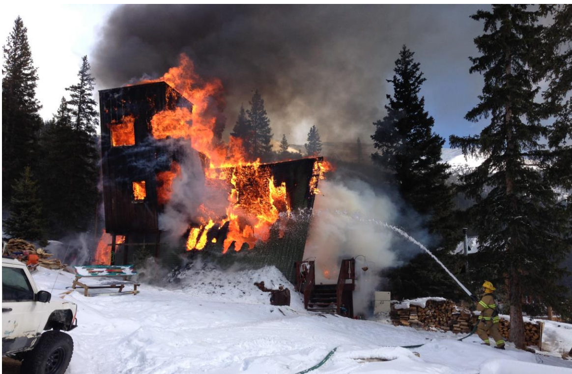
The “Tiltin’ Hilton,” a landmark A-Frame home in Montezuma, burned on Jan. 29, 2013. Although the cause was not determined, the fire appeared to have originated in the area of the wood stove. The structure was a complete loss.
